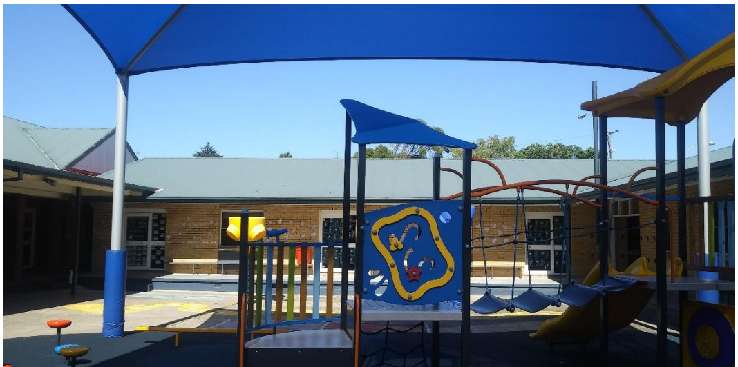
Figure 5 Existing building and play area to be demolished. Building on left to be refurbished.
