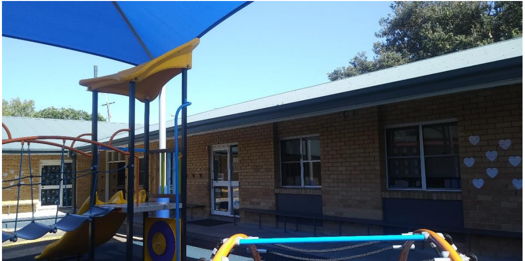
Figure 4 Existing building and play area to be demolished
