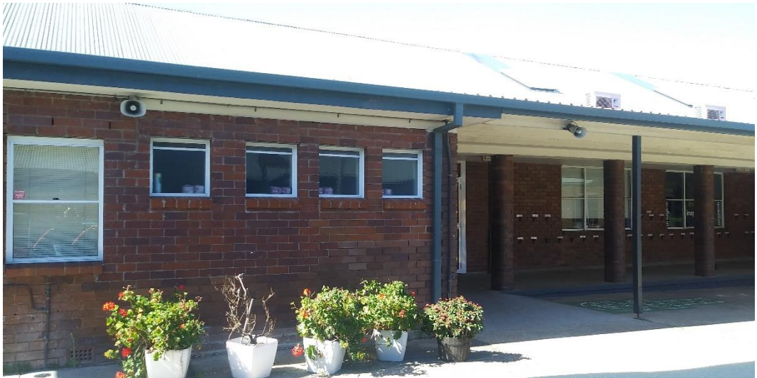
Figure 7 Existing building to be refurbished.
