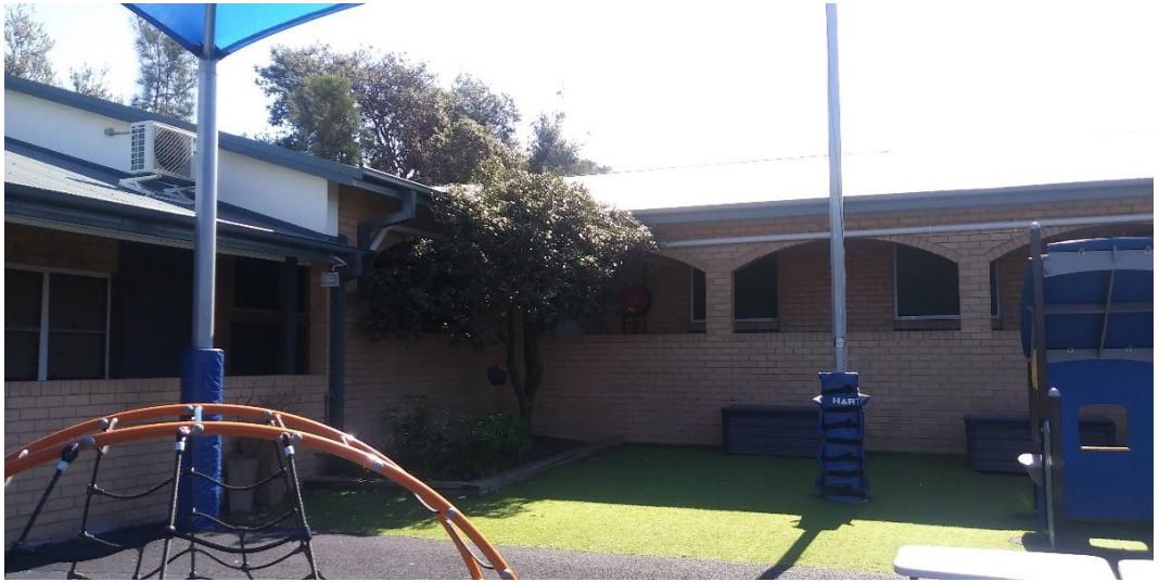
Figure 3 Existing building to be demolished
