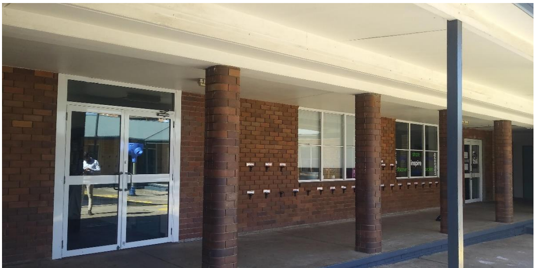
Figure 8 Existing building to be refurbished.
